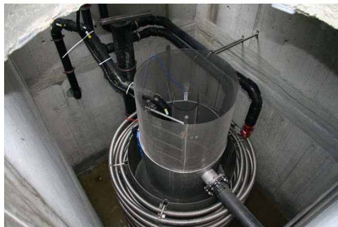
Figure 13: FEKA-tank for the heat recovery from raw sewage [Kalberer, FEKA-Energiesysteme, CH-7310 Bad-Ragaz]
